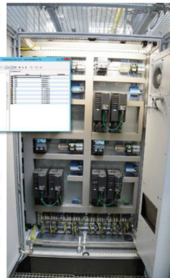
Power range in the cabinet for four booths; project structure in Engineering Base (EB)
