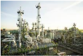
Carboxylic acid plant
